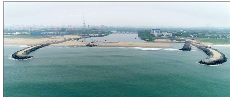
During progress of training wall : With sandbar
