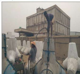
Pre-Casting of Tetrapod's in Casting Yard and Stock Yard
