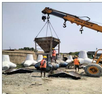
Pre-Casting of Tetrapod's in Casting Yard and Stock Yard
