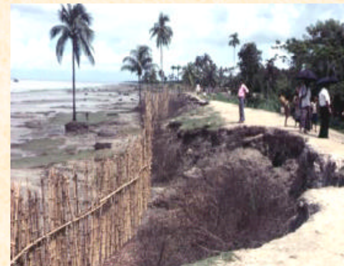
Coastal Erosion of Flood Defences
