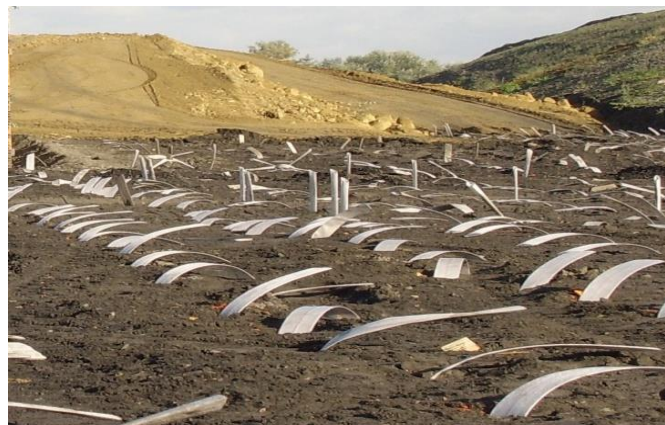
Prefabricated vertical drain as settlement reducer
