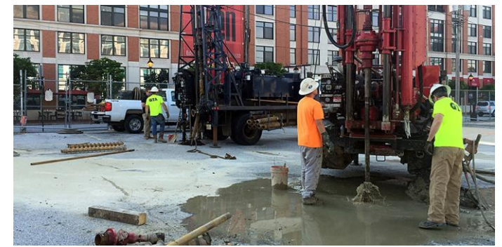
Standard Penetration Test
