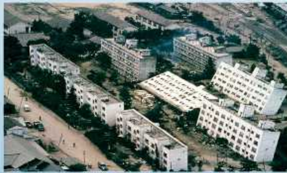
Failure of Building due to loss of bearing capacity
